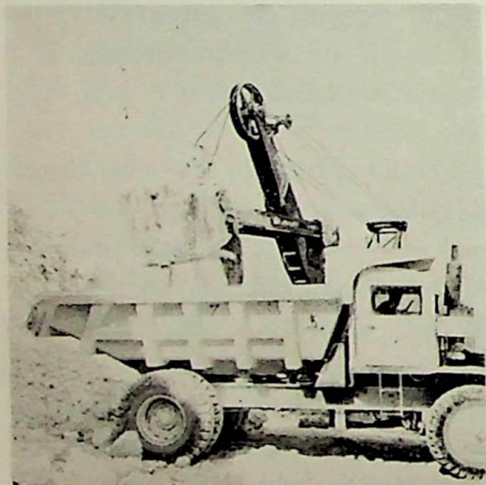
At the Lime-stone quarry
